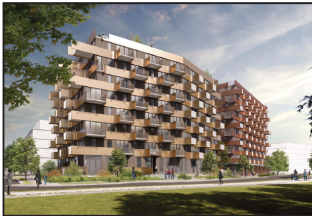
This proposed two-building, mixed-use project sits at the heart of the master-planned community of Little Mountain.
