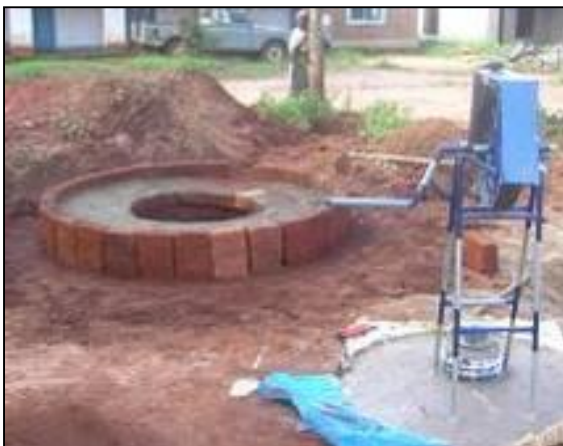
Use bricks to reduce the use of cement
