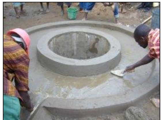
Finish the apron with a layer of cement mixture
