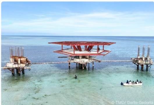
The central structure of the new ranger station is taking shape. DENR will fund the completion of the main structure, while TIEZA will fund the other two.
