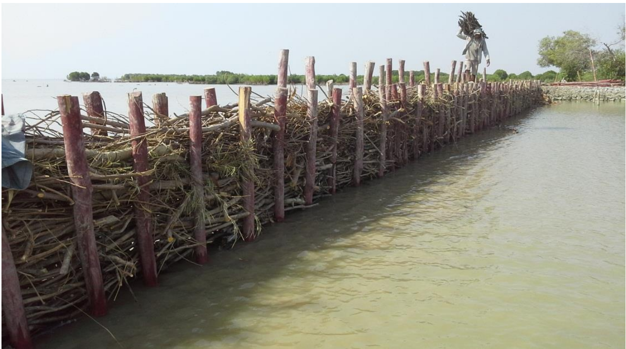
Plate 5. The process of establishment of semi-permeable structures with natural membranes perpendicular and parallel to an eroding coastline. Photo: Wetlands International and Deltares.
