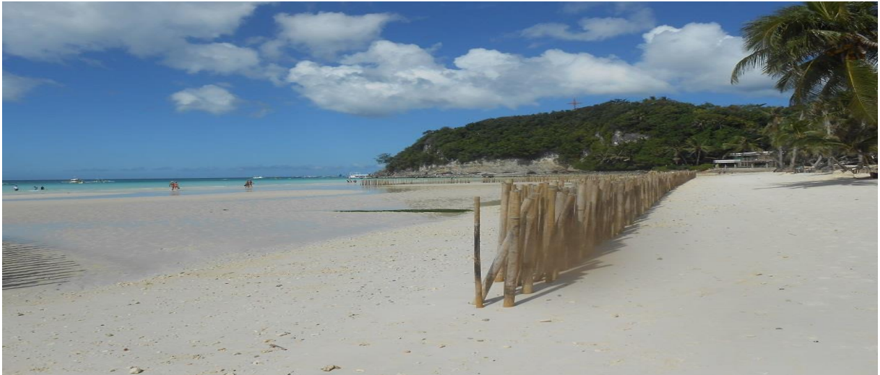
Plate 4. Experimental use of bamboo poles to halt erosion of the sandy beach of Boracay. Photo: Arne E. Jensen
