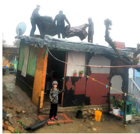
Below & right: Erik & helpers putting tarps on leaky roofs.
