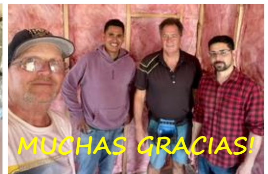
Philip shows Erik & Geovanny how to cut sheet rock.
