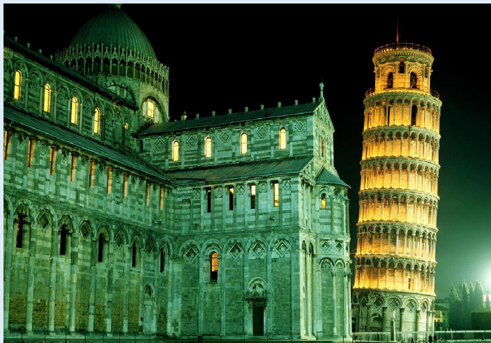
Leaning Tower of Pisa
