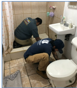
Joshua & plumber working at CJ
