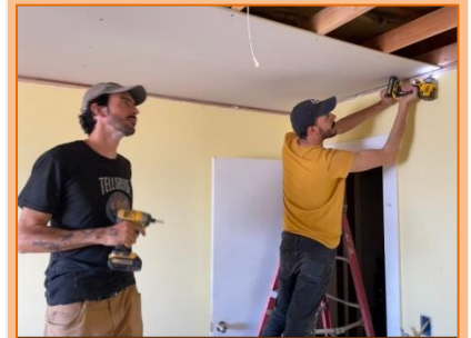
Josh & Lucas hanging drywall
