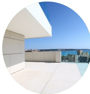
Possibility of onsite Mock Up.
