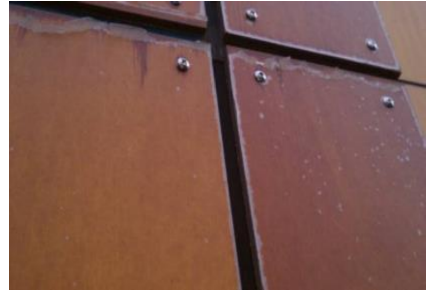
Freeze/thaw damage
