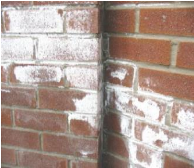
Efflorescence
