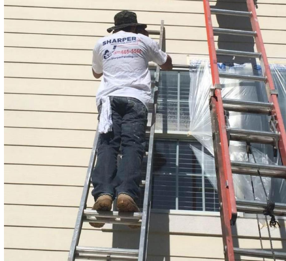
Repainting Fibre Cement – Whaaa?
