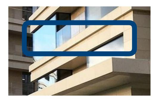
Great example showing how of combination of 3 different assemblies can help to achieve architectural idea. #1System 316 (KERF) #2 System 228 (KEIL) #3System 325 (PIN)
