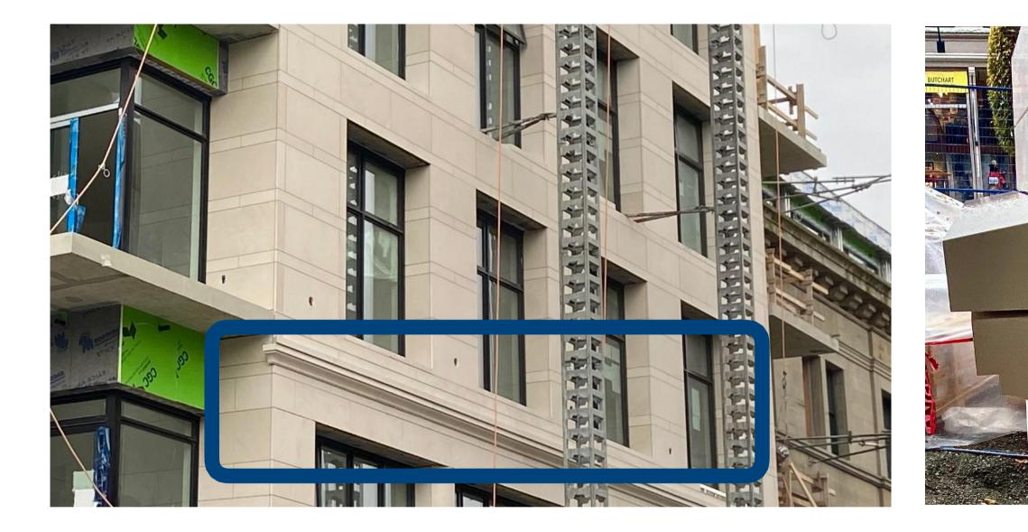
Using special shape of horizontal profiles to secure heavy cornice pieces (limestone)
