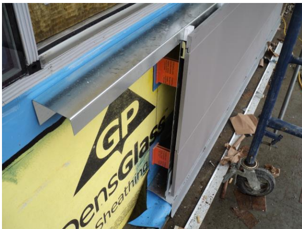
Fiberglass clips (Cascadia Clips) with vertically oriented rails
