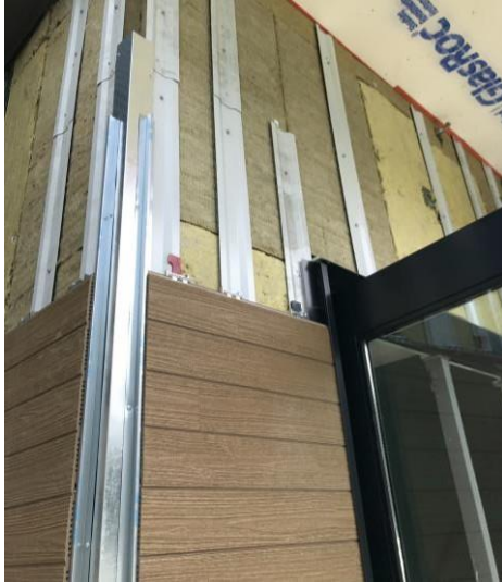
Hat channels installed over mineral wool. Extra "L" shaped metal at the corner.
