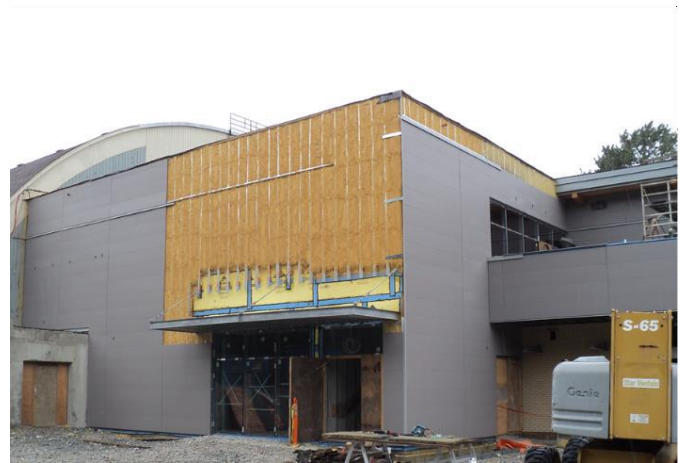
Z-girts oriented vertically with spray foam
