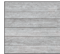
Board Formed Concrete
