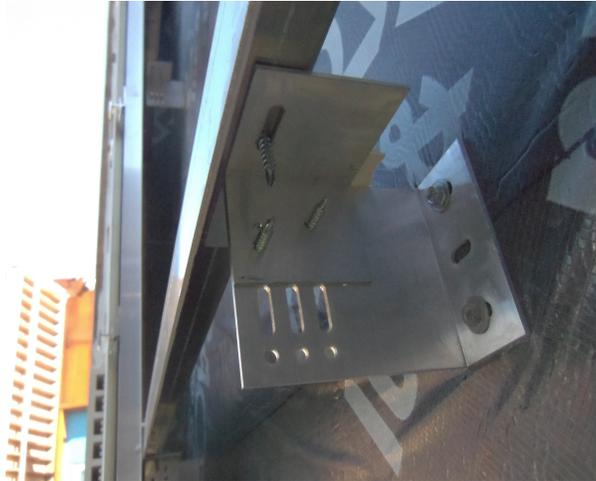
**Figure 3:** Wall bracket fastened to support T-bracket with two screws which is then fastened to the horizontal support section with two self tapping tek 1” long number 12 fasteners with a pitch of 13 and a flanged hex head that is 5/16”. This is done once for every bracket
