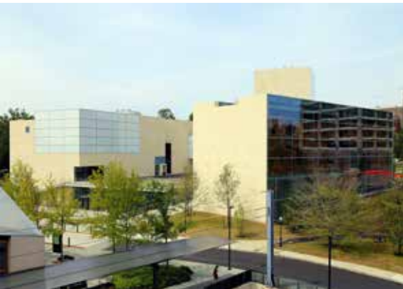
Princeton University - Lewis Center for the Arts Steven Holl Architects
