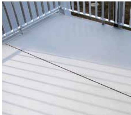
INCLINE AND PANEL JOINTS
