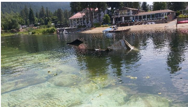
Mat install along creek; upwelling current lifted and flipped mat, mat was repositioned; Year 3
