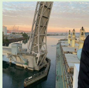
Passing through the 11 th St bridge in the Hylebos Waterway. Courtesy of Puget Sound Pilots.
