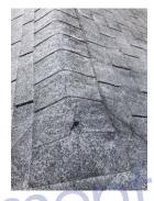
1.08.2 • The ridge shingles used to protect areas of the roof from moisture intrusion was damaged in areas. A qualified roofing contractor should inspect and repair as necessary.
