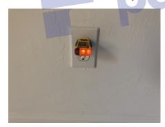
7.06.2 • Two electrical receptacles in Pink bedroom have a top plug that is not useable. Suggest contacting qualified technician to repair or replace.
