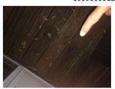
3.21.2 • Some floor joists were deteriorated at the deck rear. A qualified contractor should evaluate and repair or replace as necessary and according to current standards.
