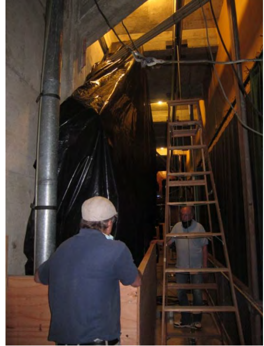
Protecting the pipework on the speaker shelf
