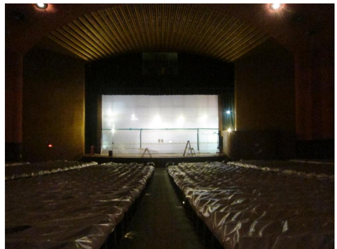
Fire curtain plastic wrapped prior to removal
