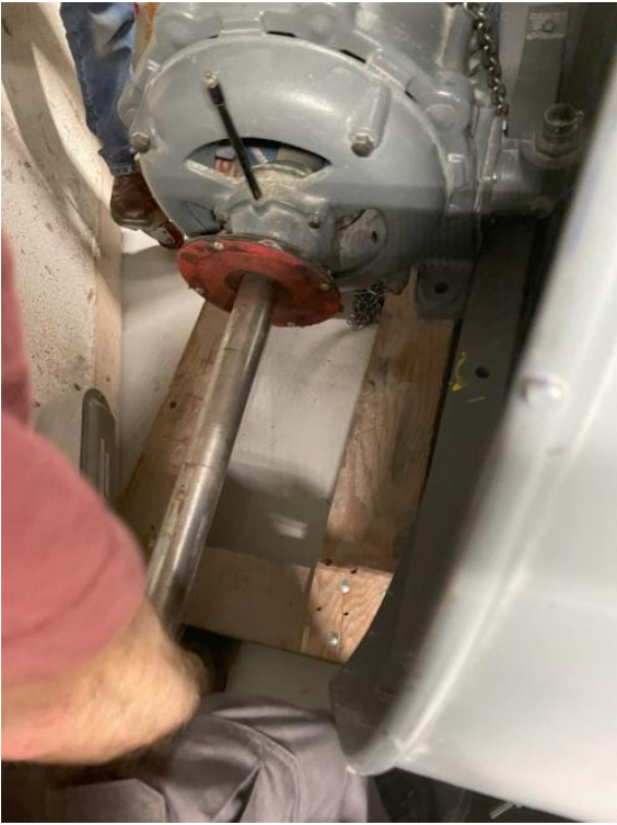
Guiding the motor into the blower shell. The shaft cantilevers some 3 feet from the motor and must be handled with great care.
