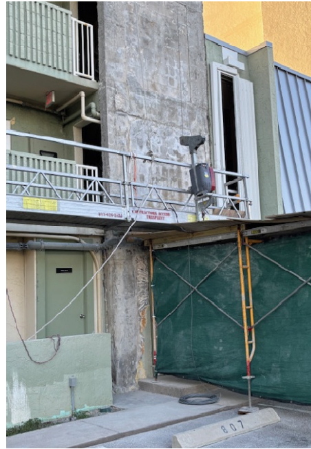
All stucco has been removed from the north tower face due to severe delaminating.
