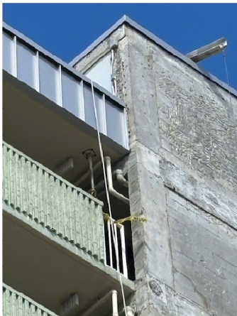
North tower stucco completely removed due to de-bonding.
