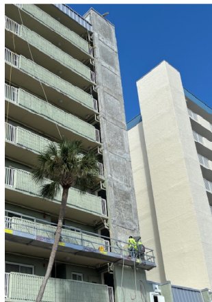
North tower stucco completely removed due to de-bonding.
