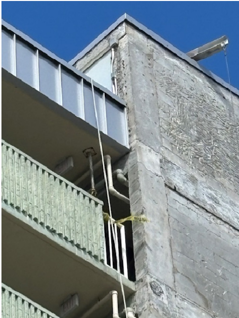
All stucco has been removed from the north tower face due to severe delaminating.
