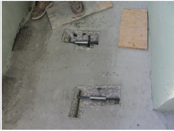
Spliced/repared cables
