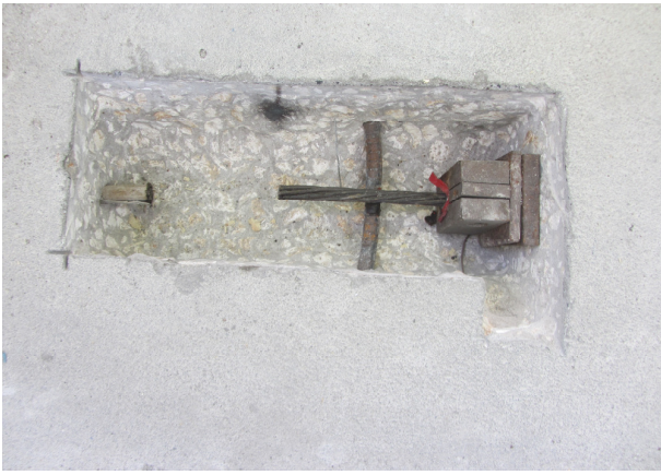
Damaged cable
