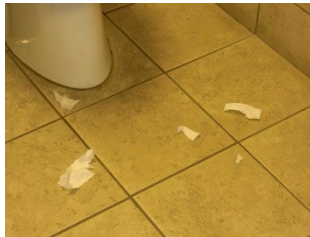
Debris on floor
