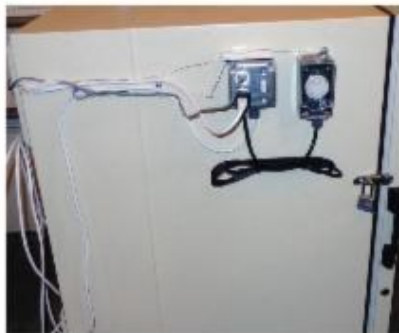
Mounted on the left-hand side of the kiln are the controls, power switch, and outlet, as well as the greenhouse controller. Note the padlock for safety.
