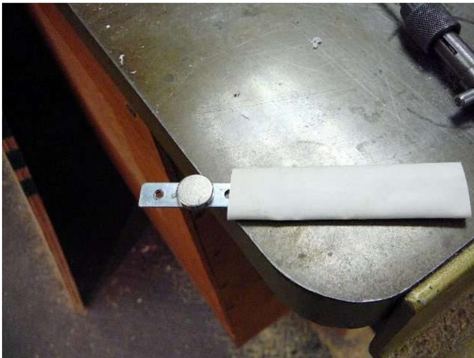
Then simple heat the tubing and the magnets are now attached to a strip that can be screwed to an item.
