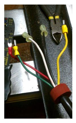
Put the connectors on the remote side of the cable. I made the red plug from some scrap rubber. Cut it to fit the conduit box and drilled a  $\frac{1}{2}$ " hole in it to accept the cable.
