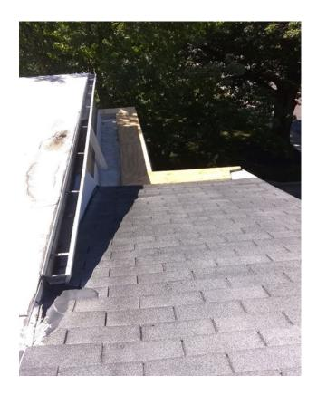
3. Hole in the roof that was under the existing shingles. This is what was found when they tore off the two layers of old shingles!
