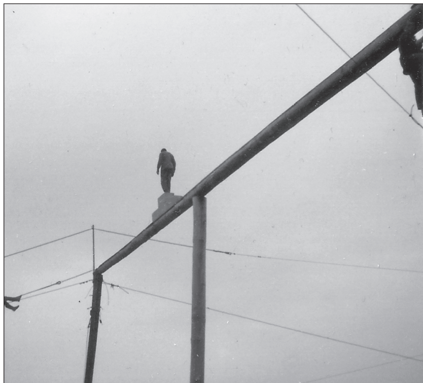
Elevated River Crossing (Chattahoochee River Valley), Ft. Benning, GA— October 1969
