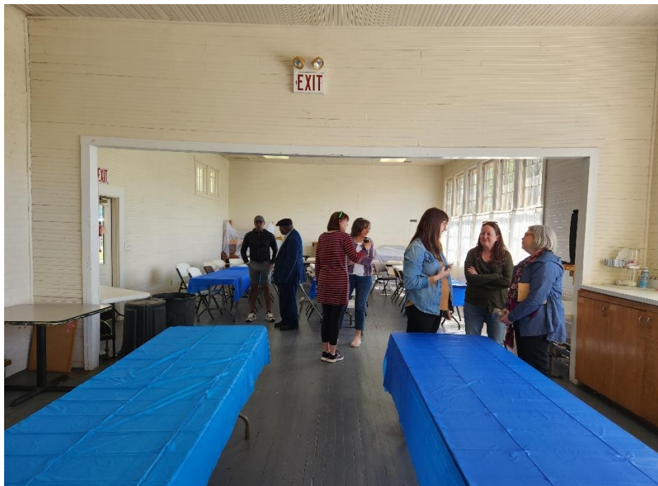
15 16 Figure 17. View looking northeast at the wall opening between the two rooms. Note, the sag at the 17 header. (PSABC 2023)
