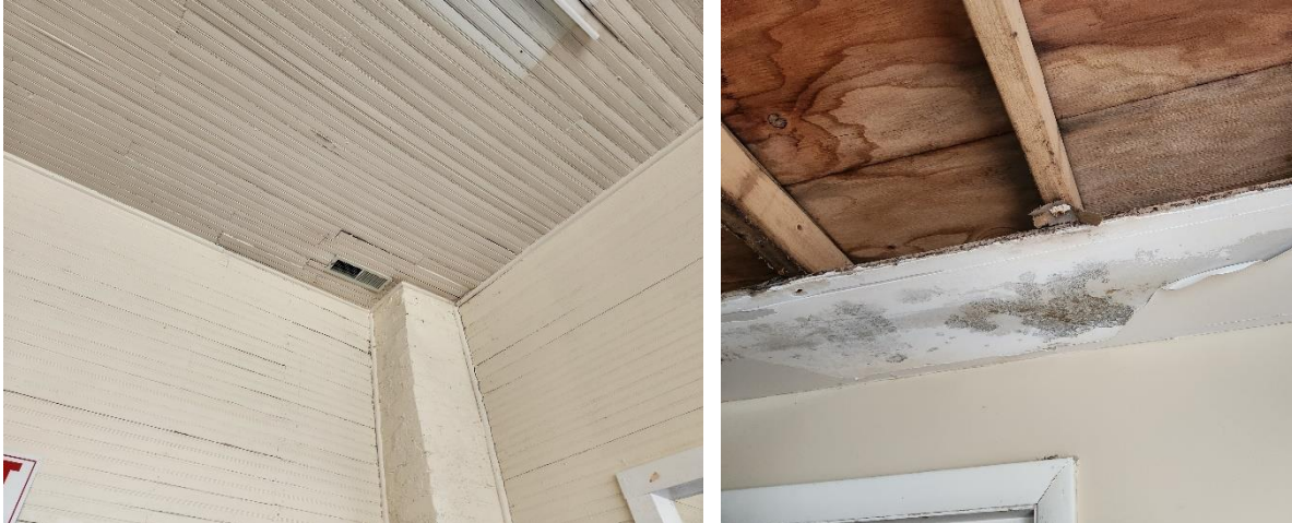
1 2 Figures 15 and 16. Left: View of the typical condition of the beadboard ceilings and walls. Right: Detail 3 view of the mold surrounding the hole in the drywall ceiling of the corridor by the restrooms. 4 (PSABC 2023) 5
