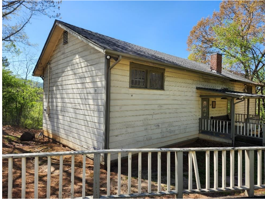
8 9 Figure 2. View of the historic Weaverville Colored School looking south at the northwest elevation (front) 10 and the northeast elevation. (PSABC 2023) 11
