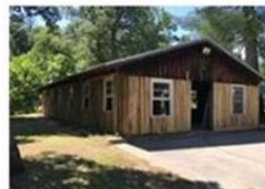
New Wood Shop - outside
