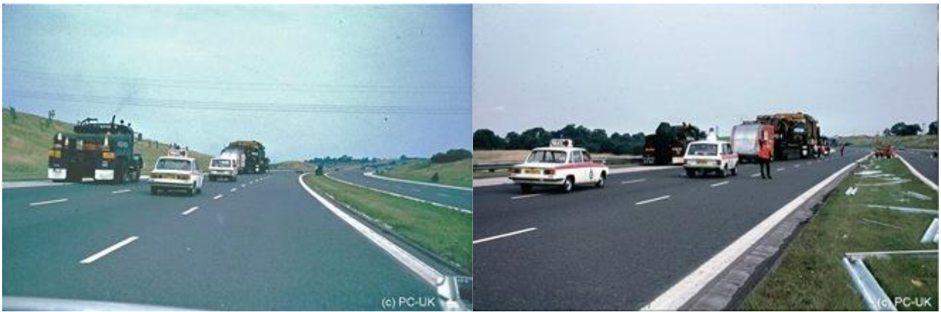
1974 Escorting a heavy transformer M1/M62. The vehicle was fitted with a skirt that was lowered and inflated like a hovercraft to spread the load on bridges. West Yorks Constabulary.
