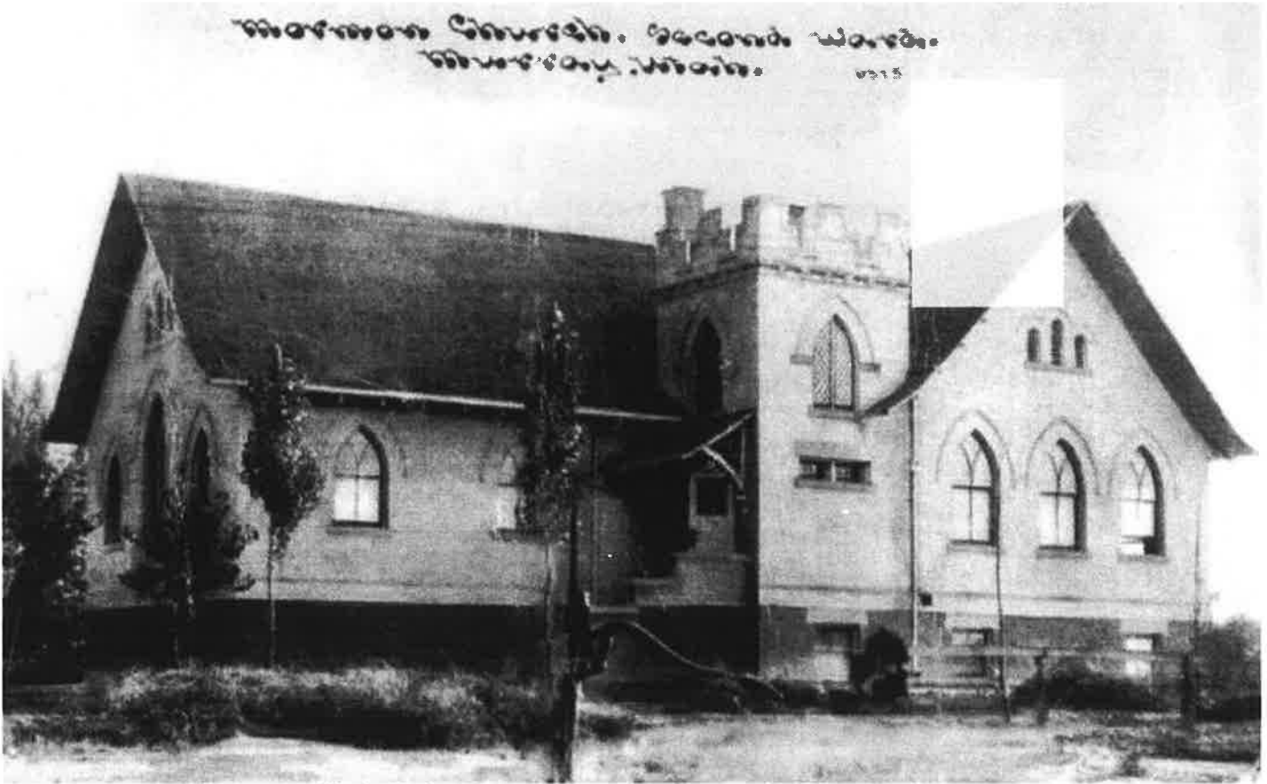
Murray, Utah 2nd & 4th Ward - Notice the hand water pump (foreground) & Horse hitching post
