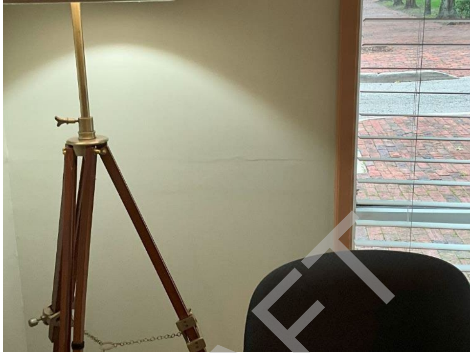
55. View of crack observed in the finish of the exterior wall of suite D-102.
