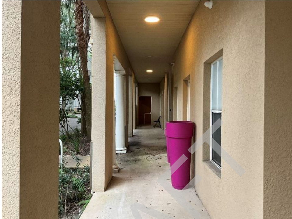
5. View of typical breezeways throughout the buildings.
