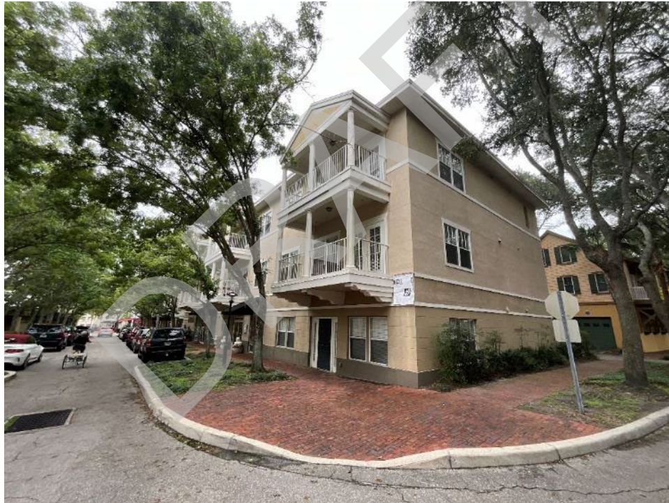
2. View of the typical front elevation of the subject complex.
