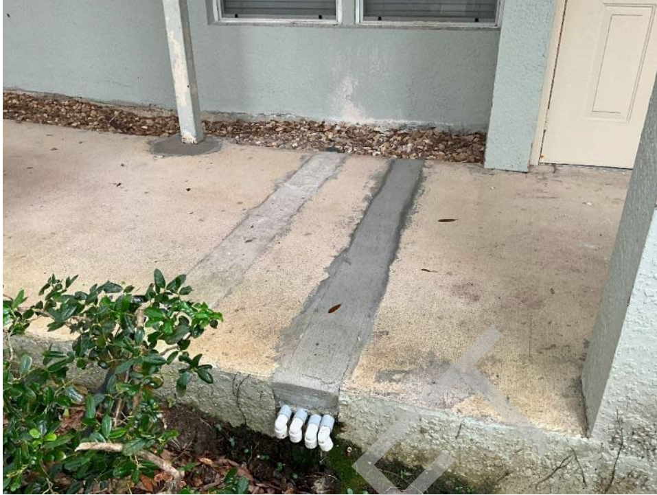
113. View of repaired slab.
