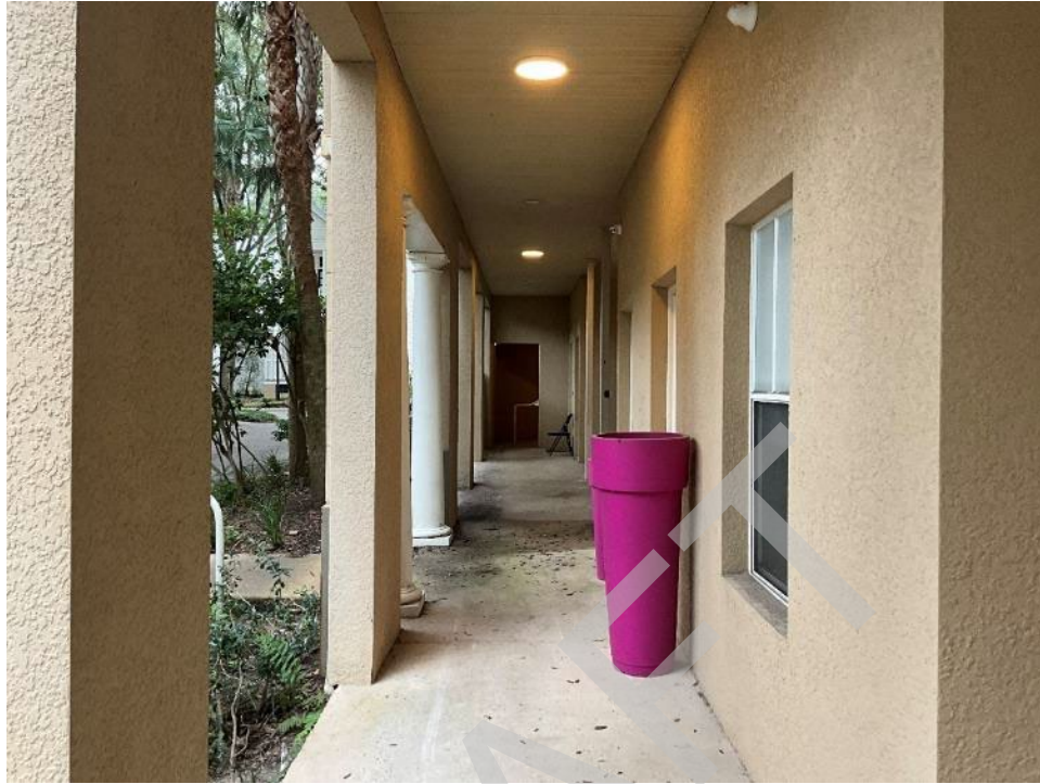
5. View of typical breezeways throughout the buildings.
