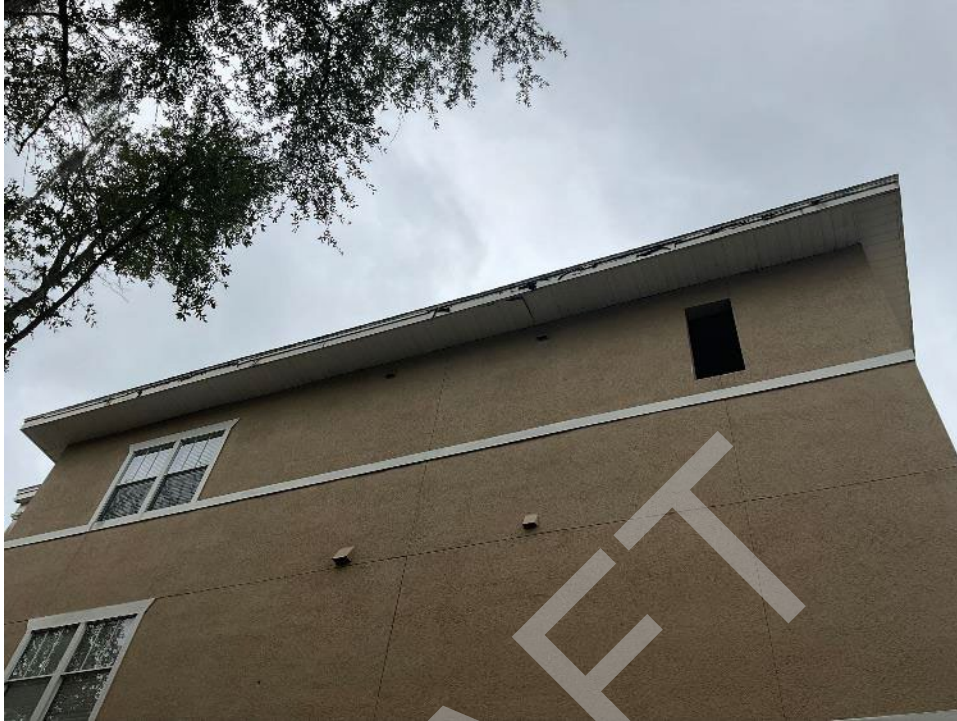
53. View of cracked section along the west elevation fascia. The fascia will need to be removed to expose the trusses for Phase II.
