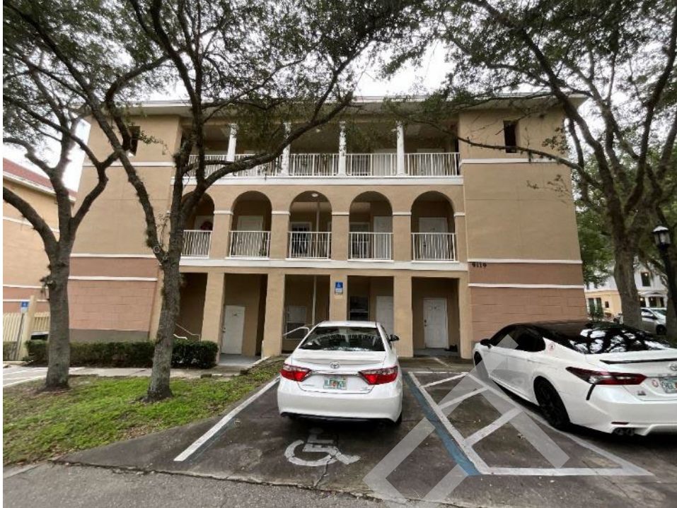
3. View of the typical rear elevation of the subject complex.
