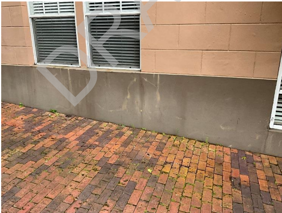
56. View of staining and cracking along the base of the walls around the building.
