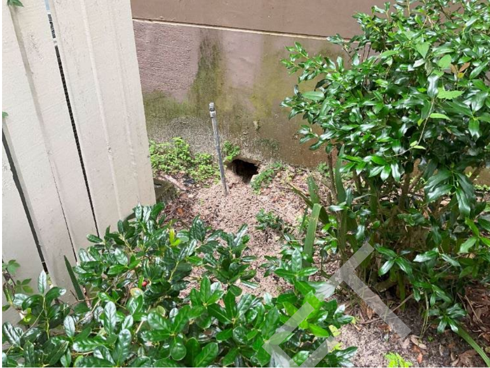
125. View of hole dug out under the building.
