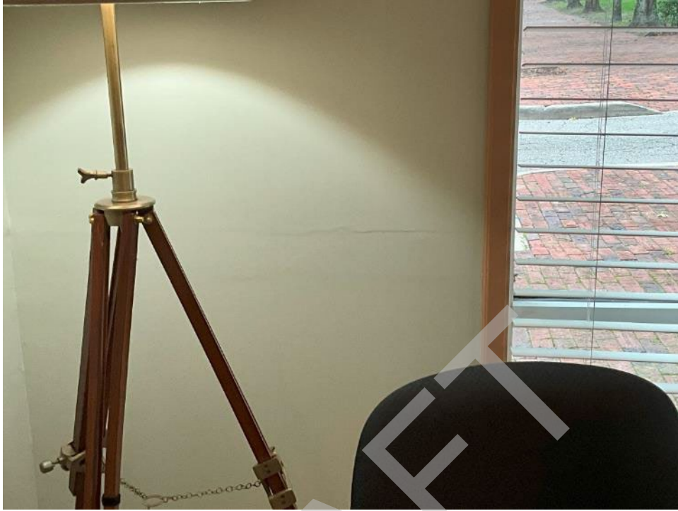
55. View of crack observed in the finish of the exterior wall of suite D-102.
