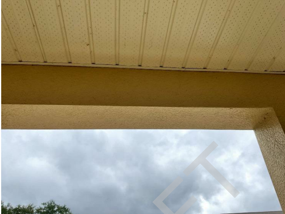
77. View of cracked section along the beam near unit G201. The stucco will need to be removed to expose the beam for Phase II.
