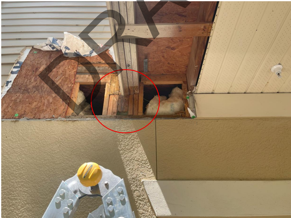
Photograph 8: View of wood blocking between the balcony joists and the CMU wall at the balcony of Unit F-202.
