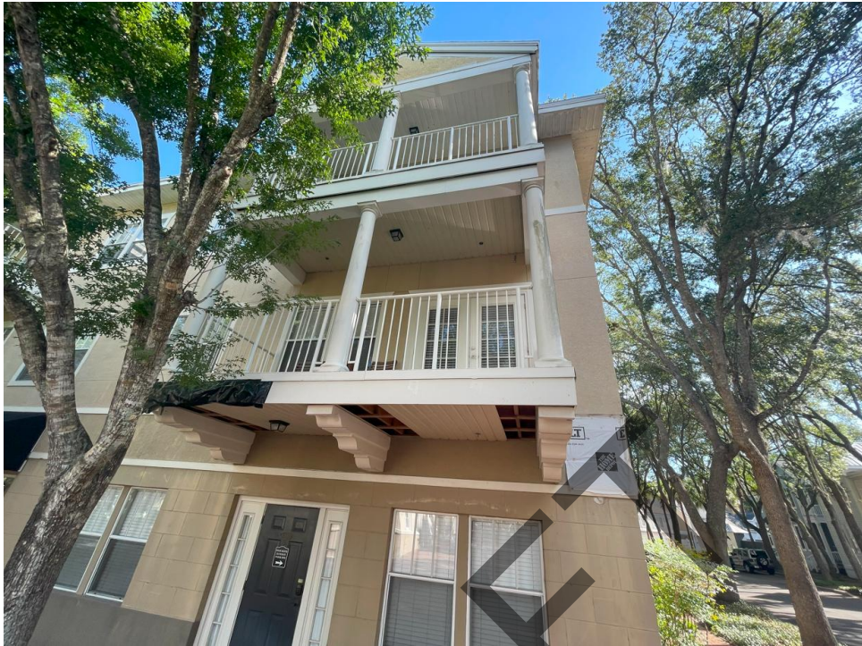
Photograph 1: View of the balcony at Unit A-201. This is a typical balcony configuration.
