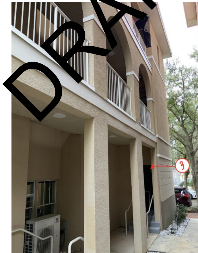
Elevation 6: View of the north elevation of Building B (West portion).
