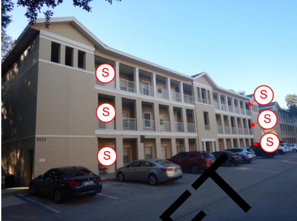
Shoring 9: View of shoring locations along the west elevation of building G.
