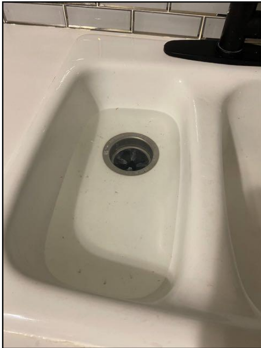
Sink backing up
