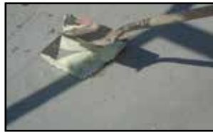
Fig. 4-3: Broken Bond
