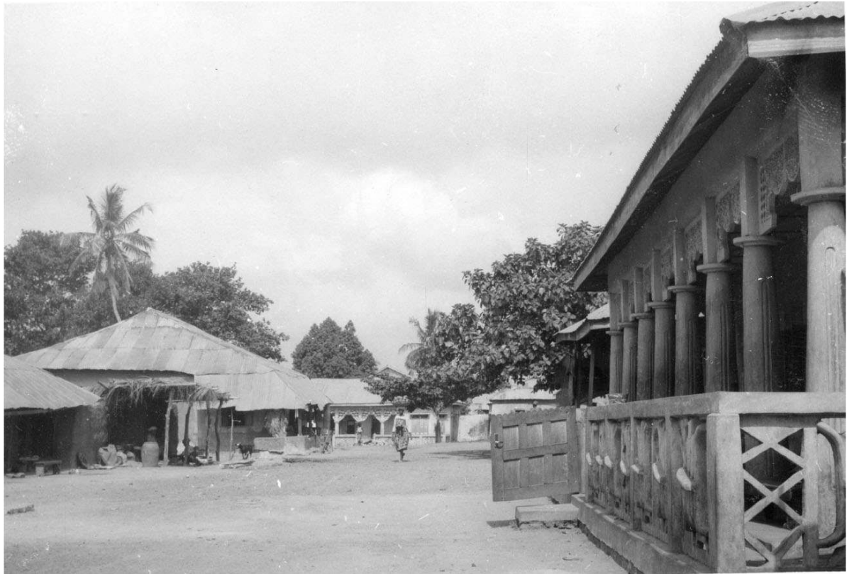
6. Decorated entrance of a compound in Oyo. Photo: Toupet, 1964, IFAN.
