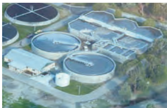
Figure 10.7 An aerial view of a sewage plant
