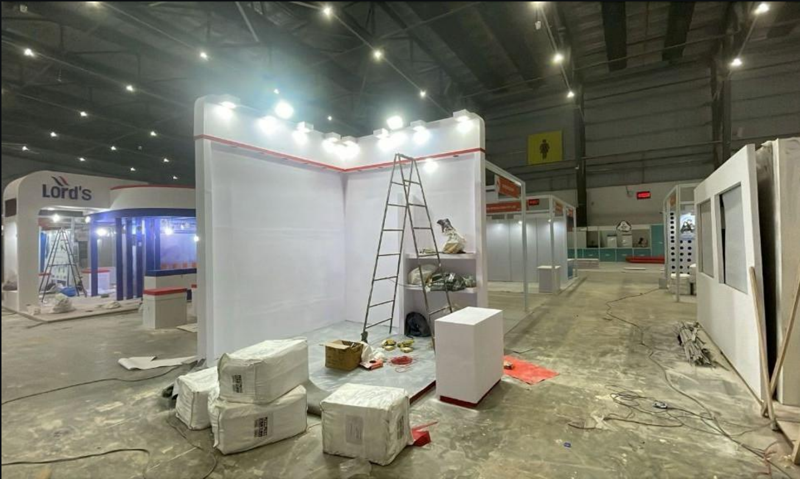
i · Booth & stage build on-site, from the ground up
