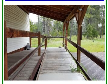
Replace the missing crosspiece on the far end of the railing in front.
