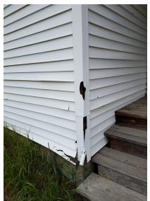
As you can see, the Grange Hall is in dire need of new siding. The old vinyl is cracked, broken, falling down, or just plain missing. Now that the new roof is
