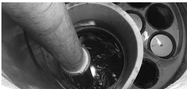
Vacuuming Sump Through MAW
