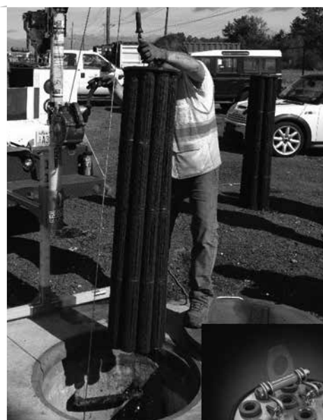
Cartridge Removal & Lifting Device
