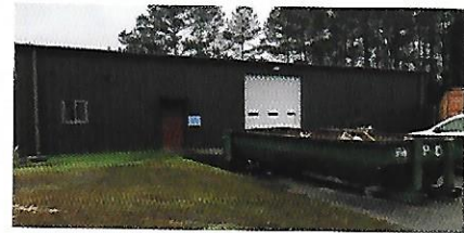
Unused warehouse, soon to transform into new training facility
