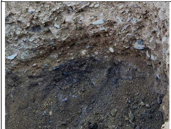
TP-3 A closer view of the subgrade soil
